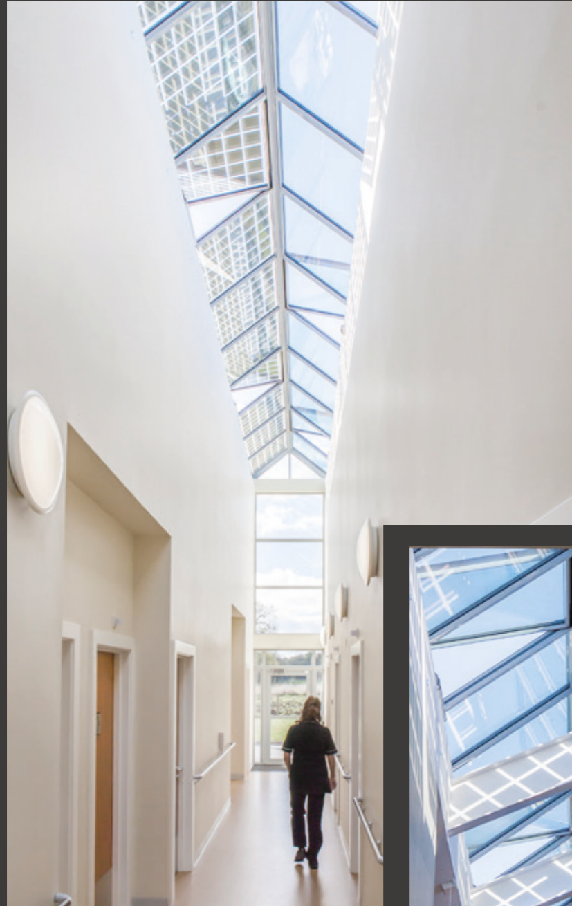
Dual pitched solution with photovoltaic panels, Ormiston, Great Britain
